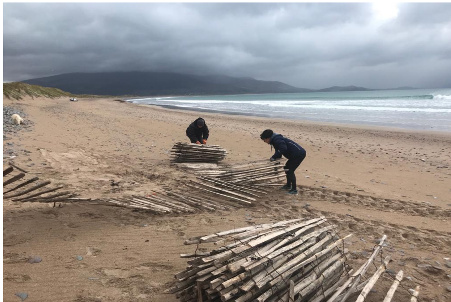
Chestnut Fencing being erected by the local community
