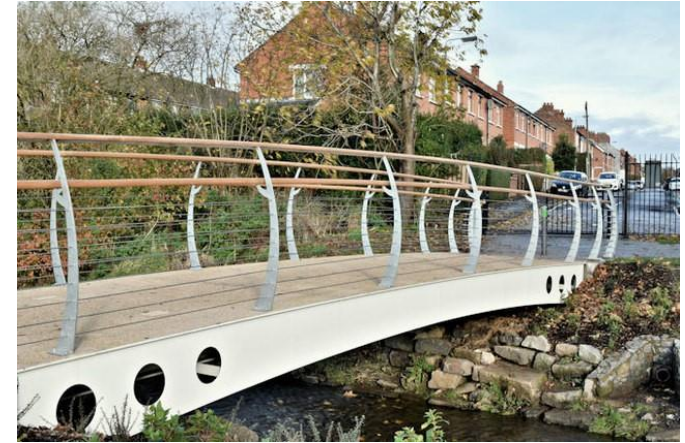
Walking bridge along the Greenway
